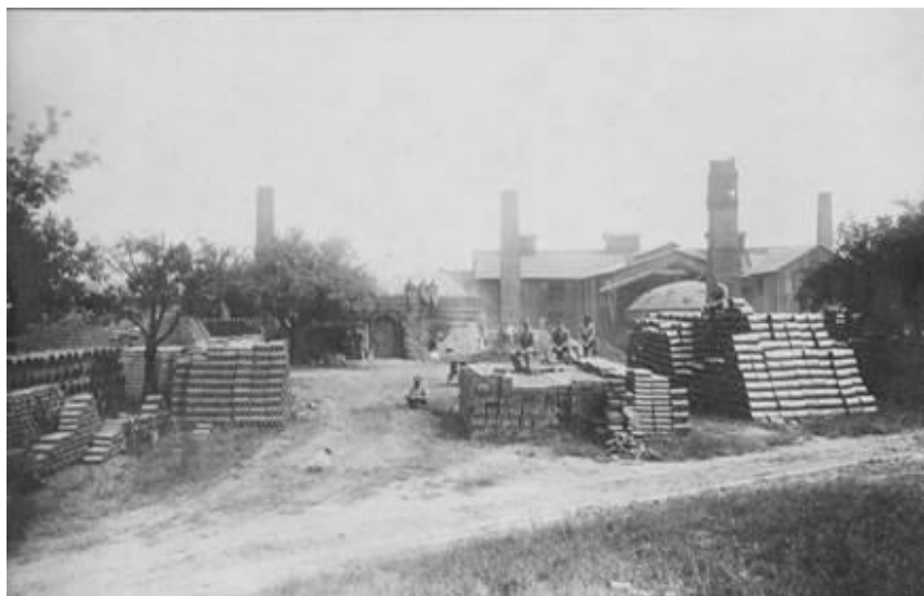
Beehive Kiln at Petty Tile Works (circa 1900). Grandpa would have been about 10
